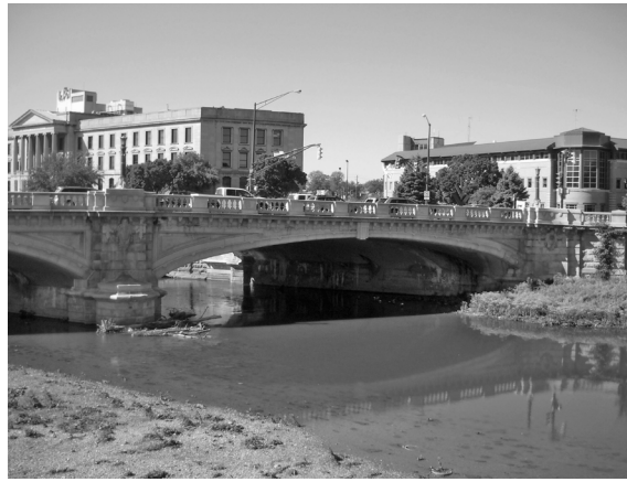
Fall Creek Bridge
