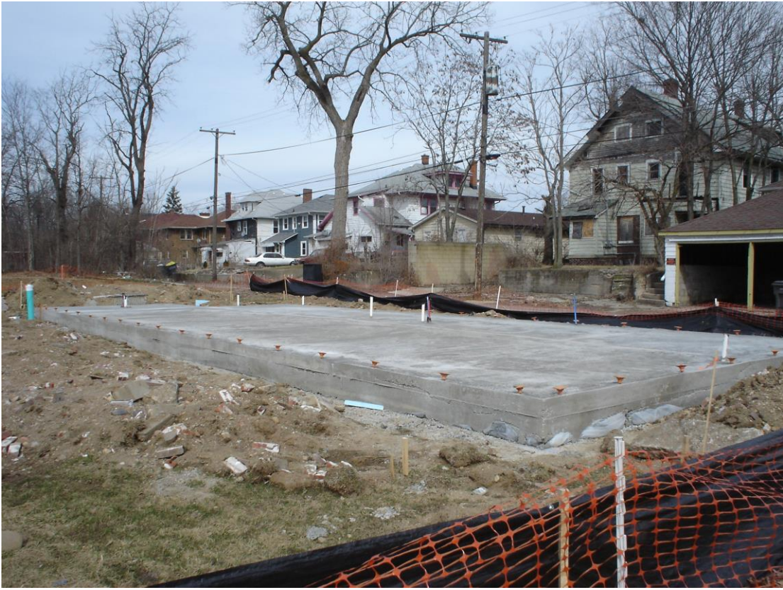
View looking northeast towards alley
